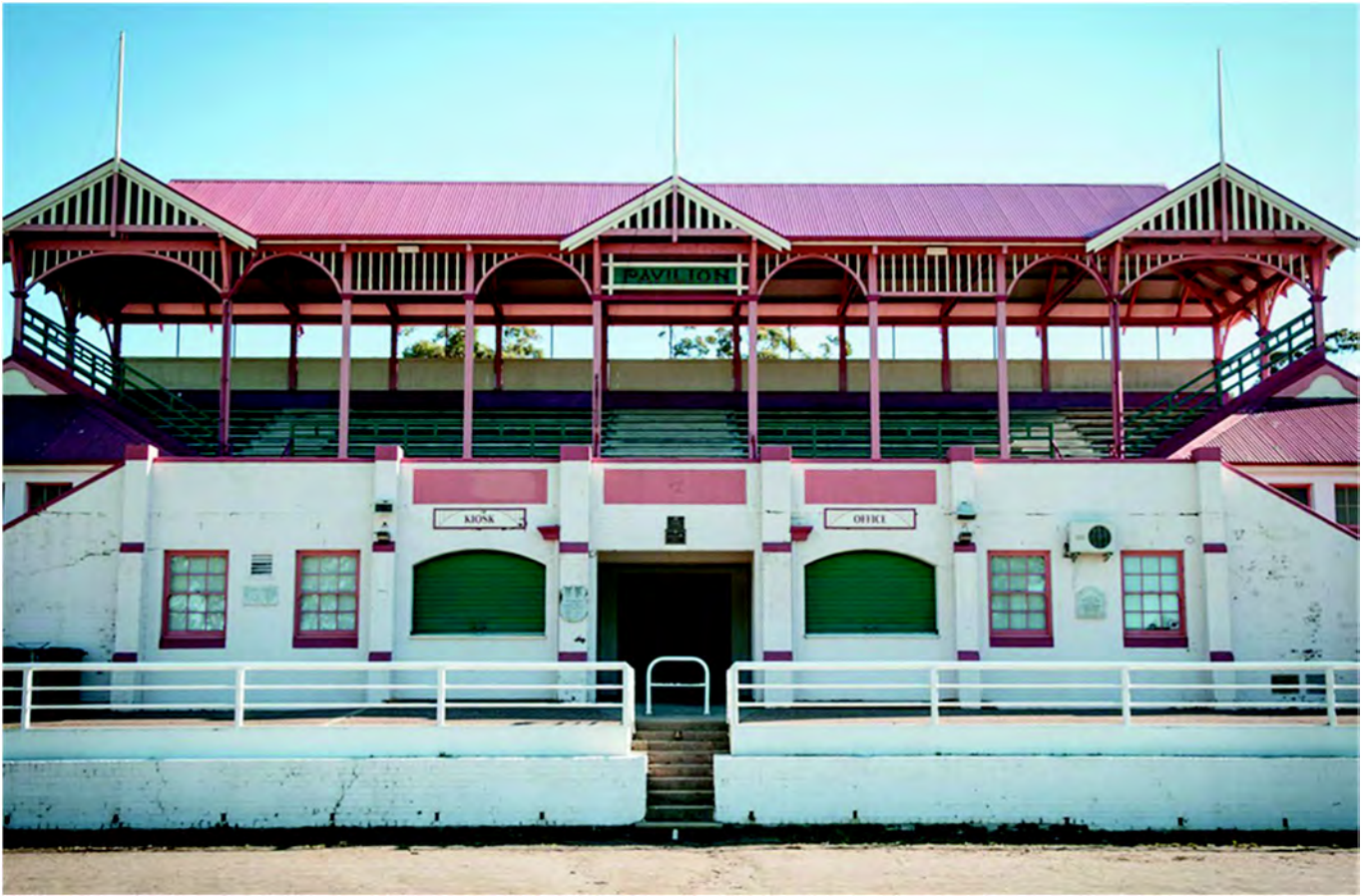
Figure 3. Nowra Showground Pavilion.
